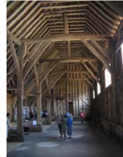
Interior of Kingsbury Barn
